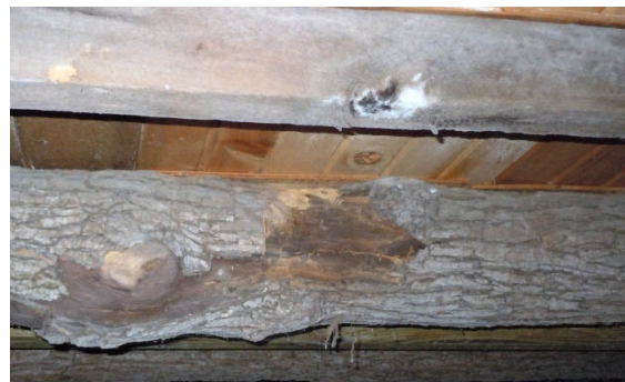
Original log joist supporting ground floor
